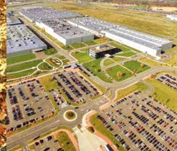
Hyundai Car Plant
